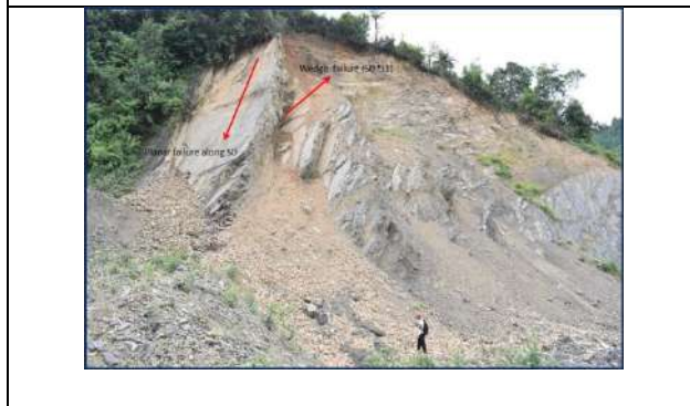
Figure 3. Planar and wedge failure of RMR15
